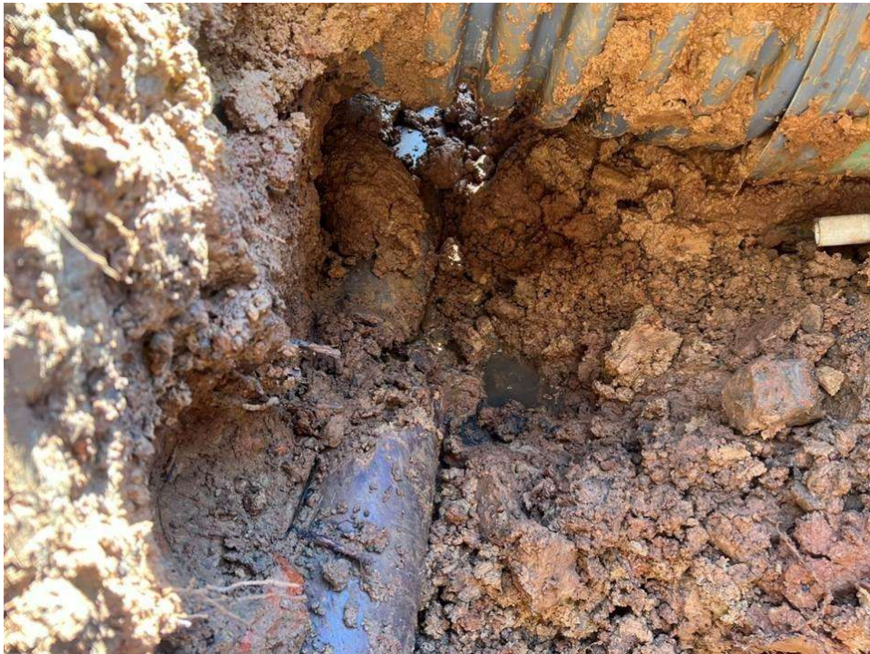
Photo 2: Fractured sanitary sewer line directly under the location of a new corrugated stormwater pipe.
