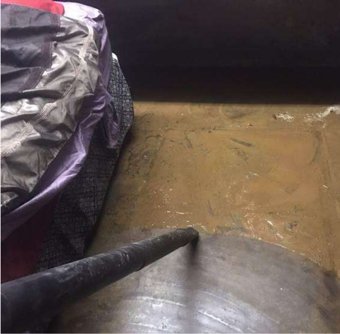
Photo 8: Vacuuming the mud from the basement.
