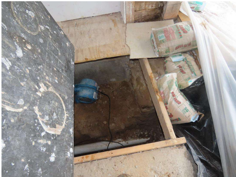
Photo 10: Rectangular opening leading to the crawlspace with a PVC sanitary sewer line visible.
