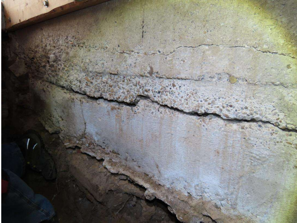
Photo 11: Longitudinal fracture approximately down the middle of a concrete beam where there was an unusually high concentration of exposed aggregate.
