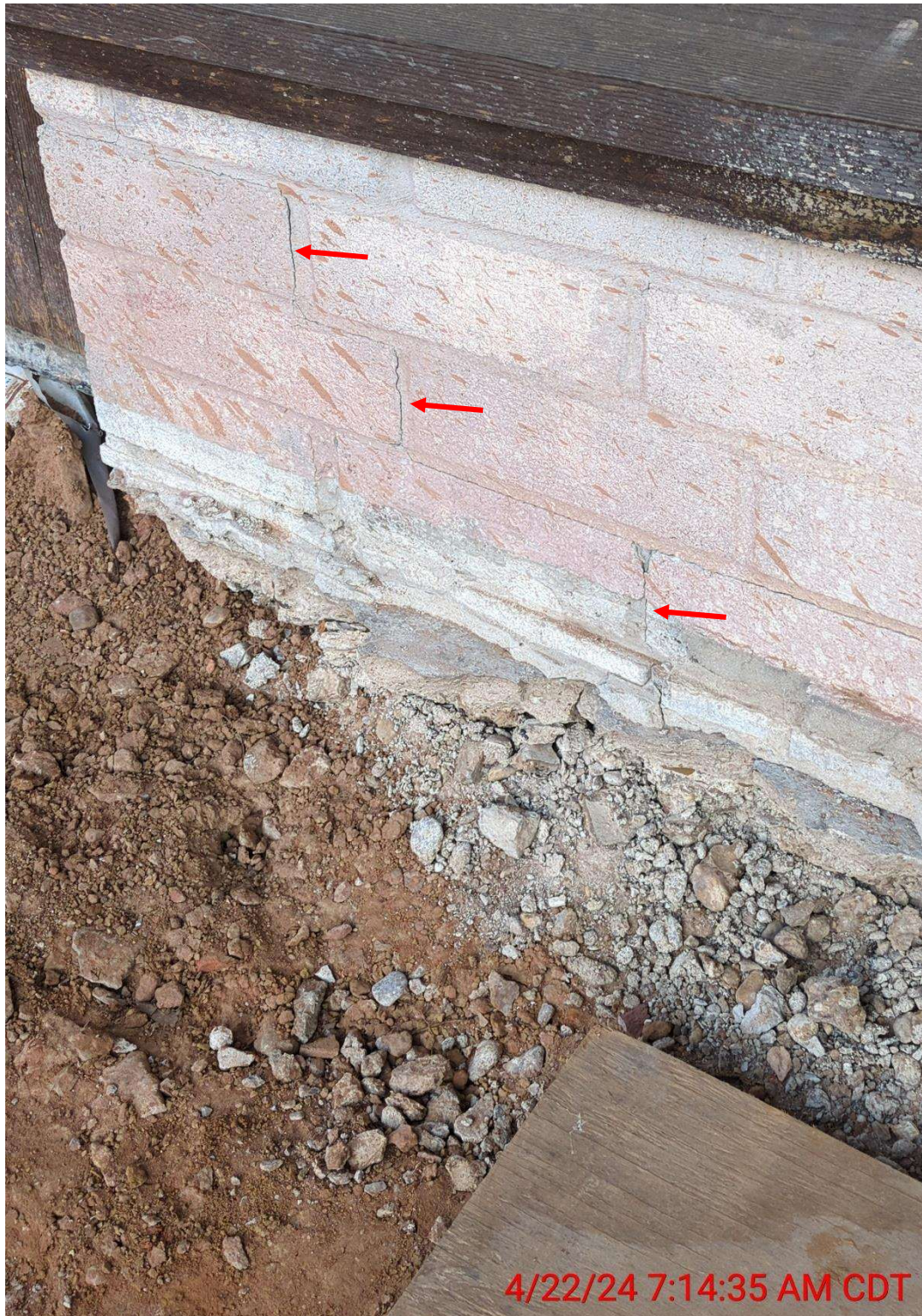
Photo 2: North side of the brick storefront wainscot, having been saw cut and chipped, with a distinct line indicating the location of the finished walkway surface. Note the fine stair-step cracks (indicated).
