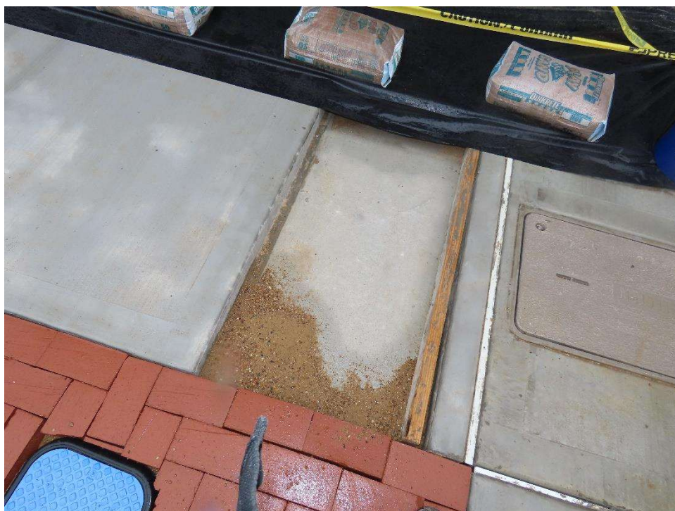
Photo 4: Accumulated dirt and sediment in a concrete trough not yet filled with brick.
