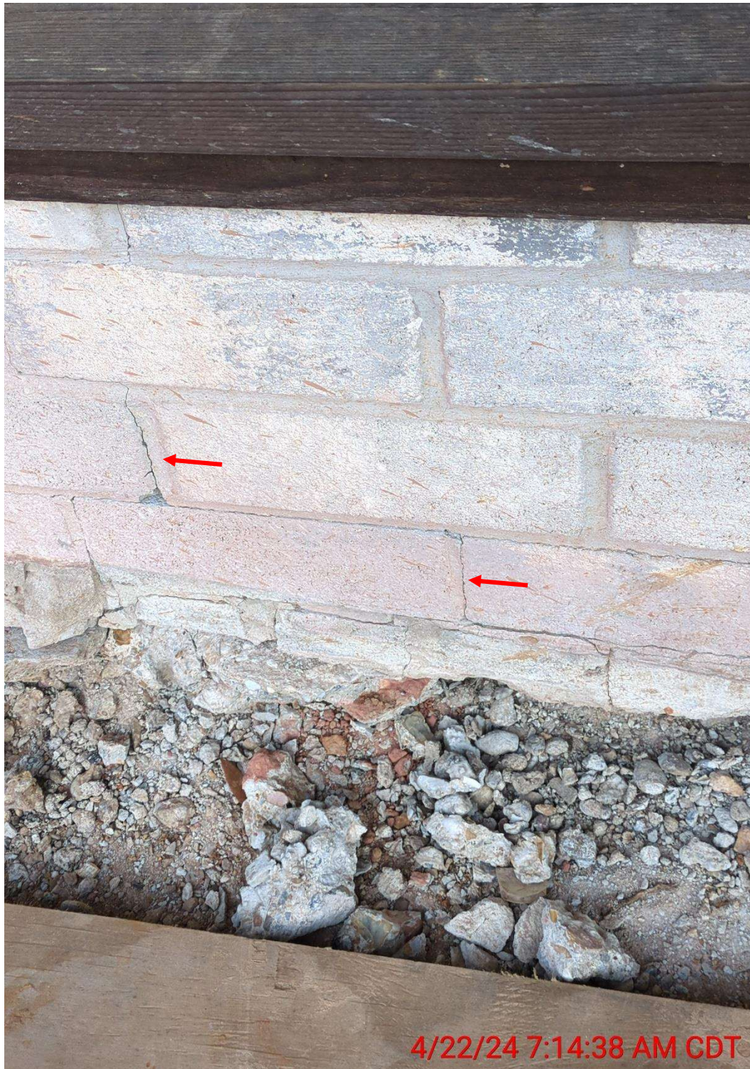
Photo 3: North side of the brick storefront wainscot, having been saw cut and chipped, with a distinct line indicating the location of the finished walkway surface. Note the fine stair-step cracks (indicated).
