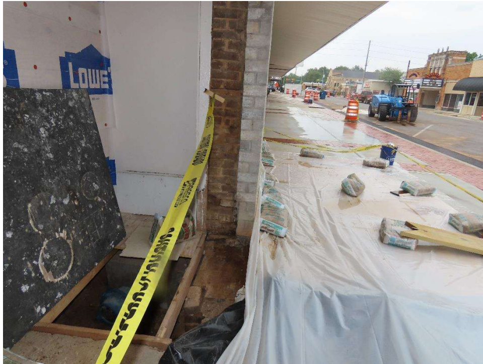
Photo 5: Remaining veneer brick and structural brick behind it at the north edge of the entryway.
