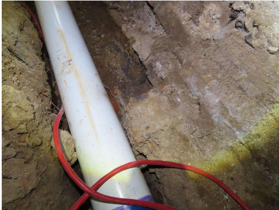
Photo 17: New PVC pipe in the crawlspace.
