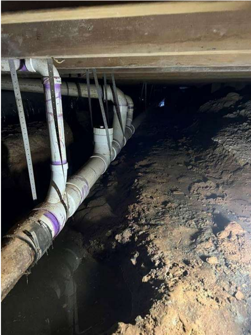
Photo 6: Flooded crawlspace under the newly installed PVC sanitary sewer line.
