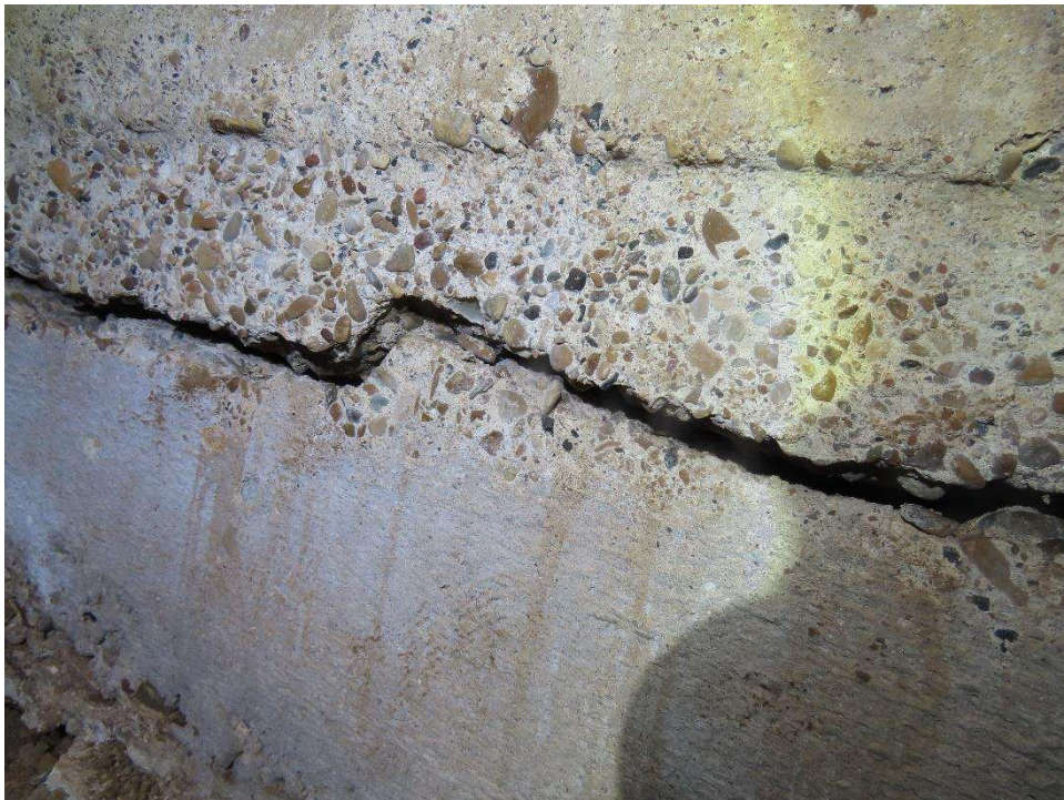
Photo 12: Close-up of the condition depicted in Photo 11 , showing the rounded edges of the fracture.
